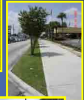
Wider sidewalks, new sod & trees in the ROW with irrigation installed.
