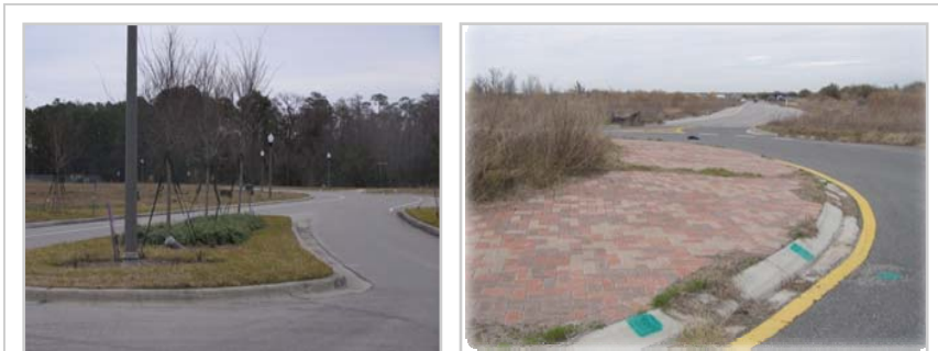
Examples of unused infrastructure in the Horizon West area
