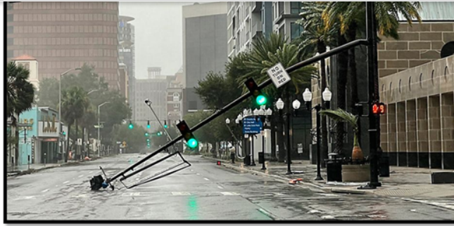
A stoplight pole at Livingston Street, blown down by Hurricane Ian winds, rests on Orange Avenue in Downtown Orlando. (Willie J. Allen Jr./Orlando Sentinel via AP)
