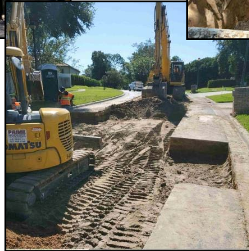
Installing roadway base
