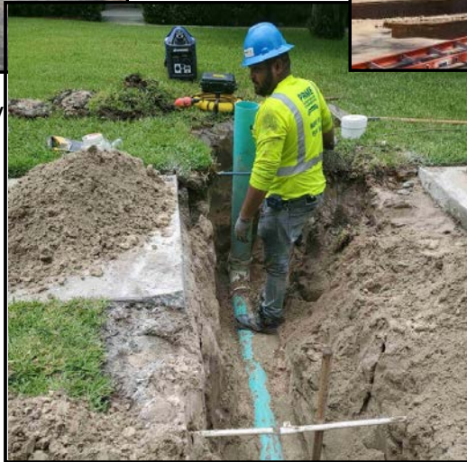
Installing sewer lateral
