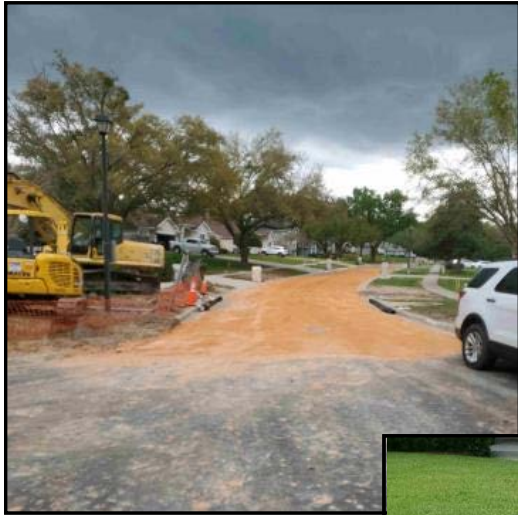
Installing roadway stabilization
