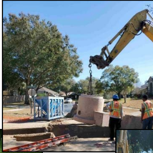
Installing manhole
